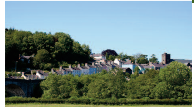
The familiar view of Bridge Street, Llandeilo from across the River Tywi. The prominent and many coloured frontages to the houses defines this entrance gateway into the town and reinforces the sense of place.
