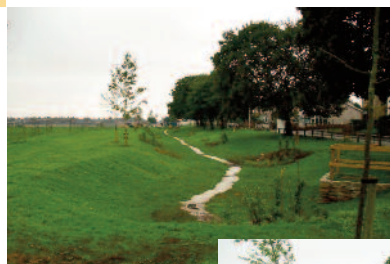
The use of a swale as part of a SuDS, Llanelli.
