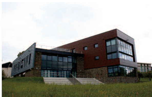
Quality modern design at the new teaching and learning building at the University of Trinity Saint David in Carmarthen.
